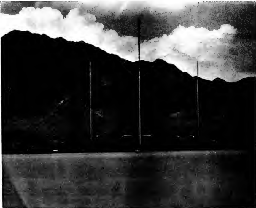
The great Radio station of the Federal Company at Ko ko head, Honolulu. The masts are 600 feet in height.
